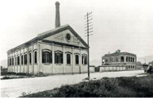
CLP's first power station at the junction of present-day Chatham Road and Princess Margaret Road.
