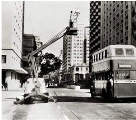
Repair of street lights on Nathan Road in the 1960s
