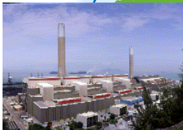
Castle Peak Power Station
