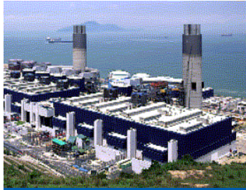
Black Point Power Station
