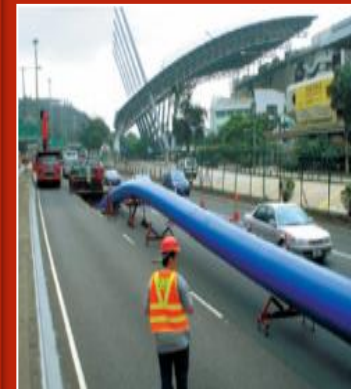
Reprovisioning of Water Mains
