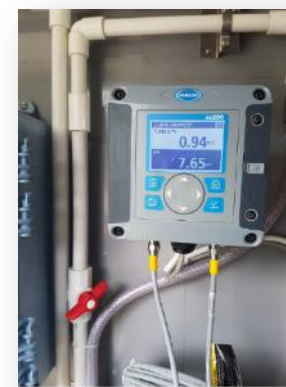
Water Quality Sensors, e.g. chlorine, turbidity
